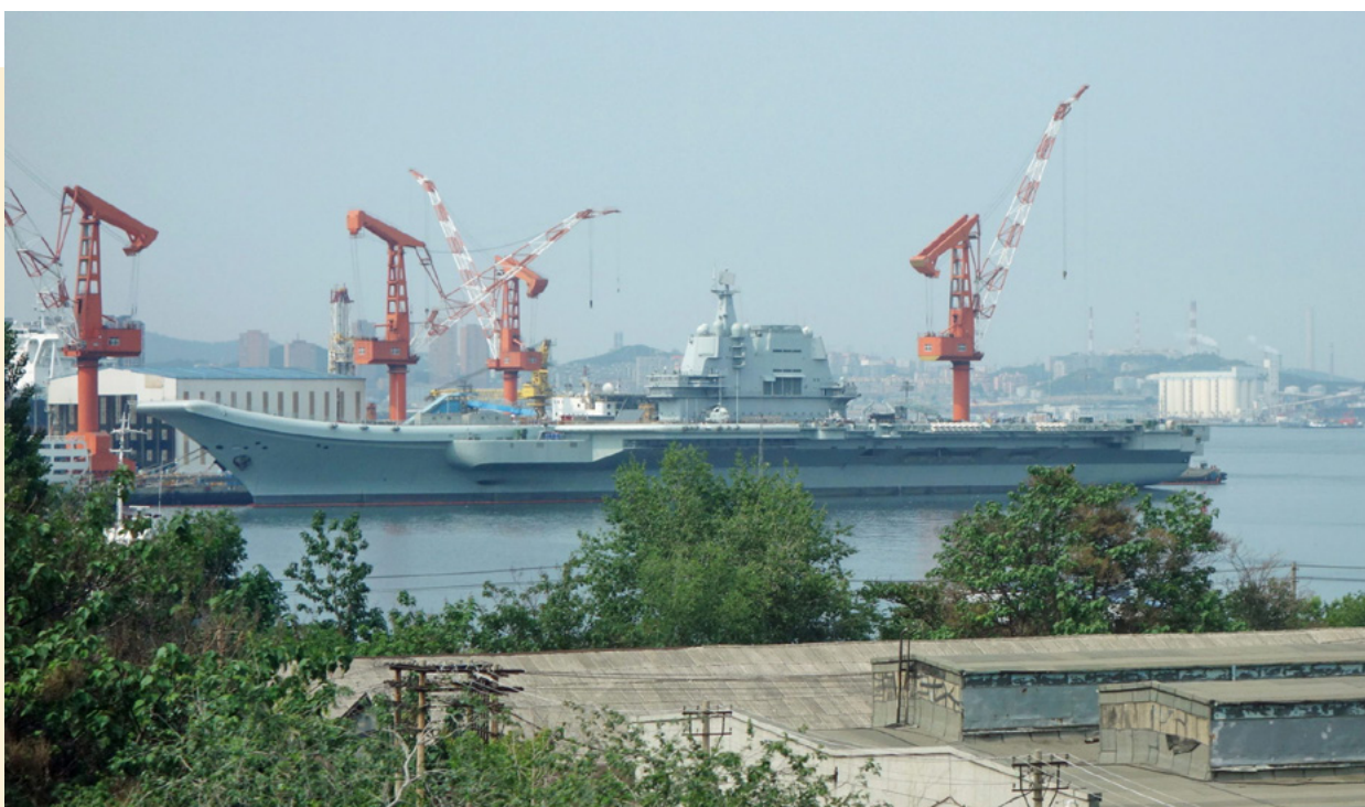
The first domestically-made aircraft carrier of the Chinese Navy under construction, 17 June 2019.
